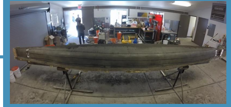
Figure 18: Apply Post-Tensioning
